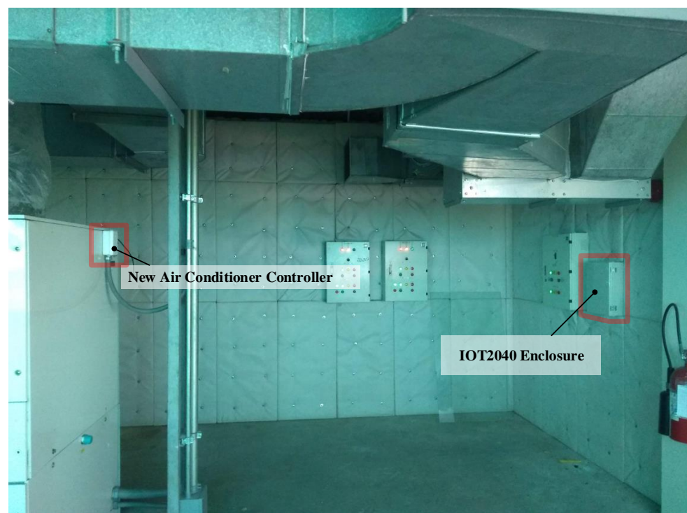
Figure 6. Air conditioning unit with IOT2040 installation.
