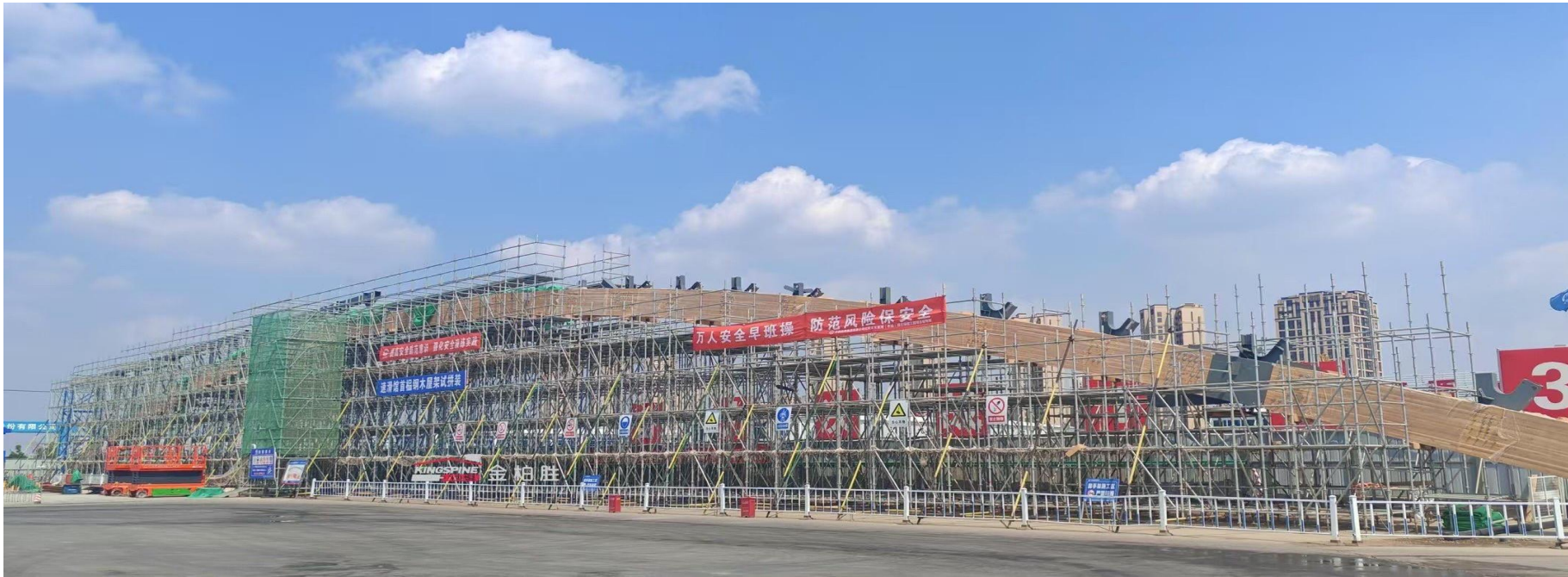
Speed skating stadium (under construction)
