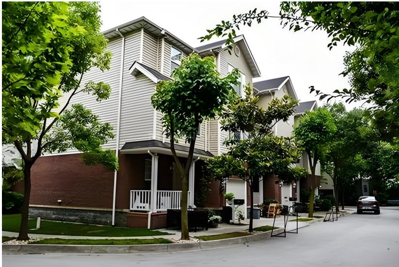
Residential construction Suzhou City Light frame timber construction
