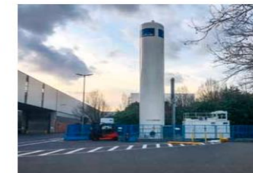
Fuel cell forklifts fueling station
