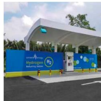
Refueling station in Sarawak (Malaysia)
