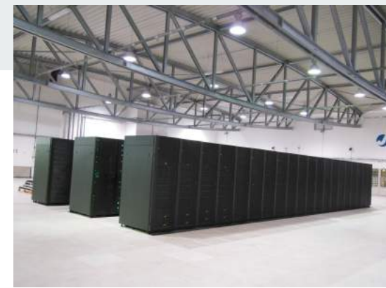
20PB SpectraScale storage at Jülich SC
