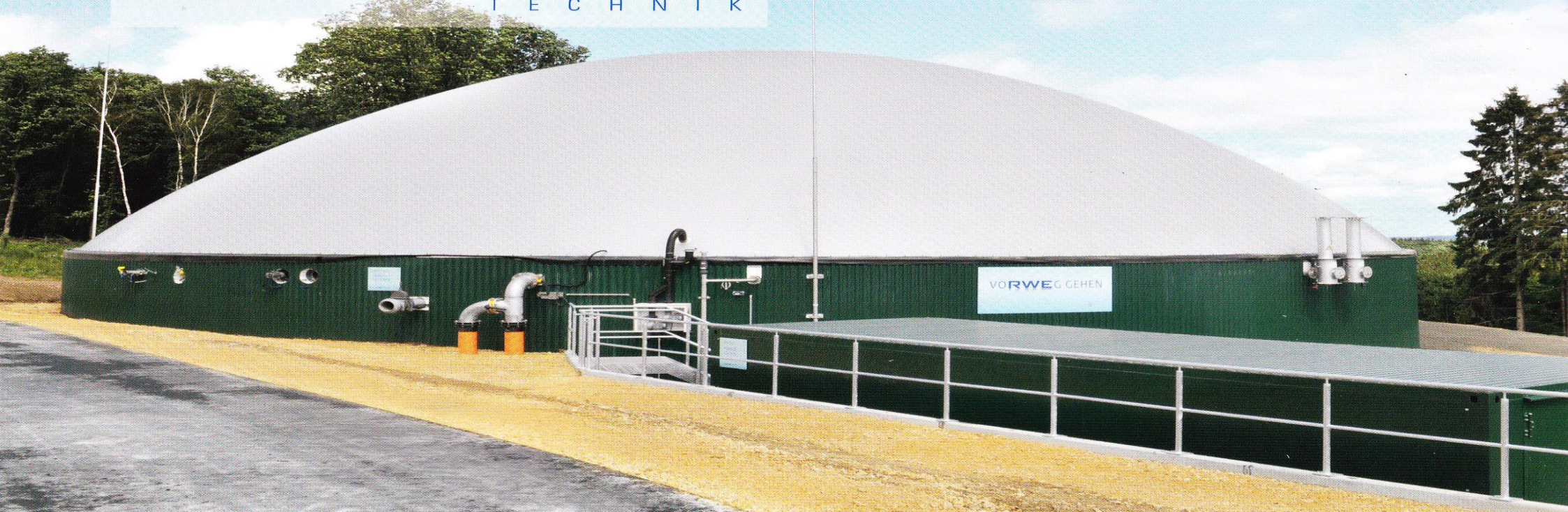
Biogas storage tank of the pilot project 'Smart Grids' operated by RWE Germany in cooperation with the Federal Ministry of Economics and Technology in the Eifel region.
