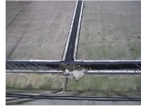
Figure 16 Undestroyed surface waterstop system
