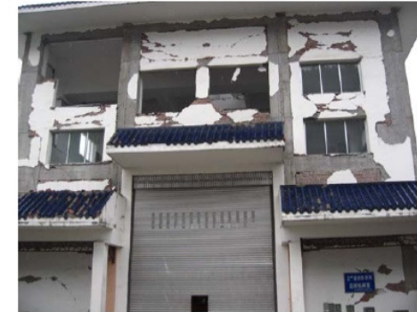
Figure 17 Damaged gate chamber structure of spillway tunnel
