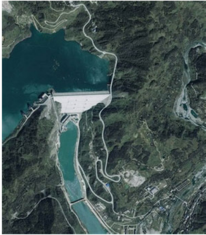
Figure 10 Satellite Image of Zipingpu CFRD before the quake
