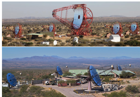
Figure 4: Top : The H.E.S.S telescopes located in Namibia. In the foreground the 28 m diameter HESS-2 telescope is seen. In the background one of the four 12 m diameter HESS-1, Below : Three of the four 10 m diameter VERITAS telescopes located in Arizona. telescopes.
