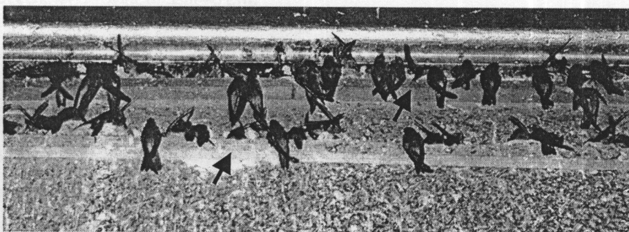
Figure 5.2. The supporting wood (dark arrows) attached on the smooth wall under the ceiling in the sacred building of Suthiwatwararam Temple, Samut Sakhon Province.
